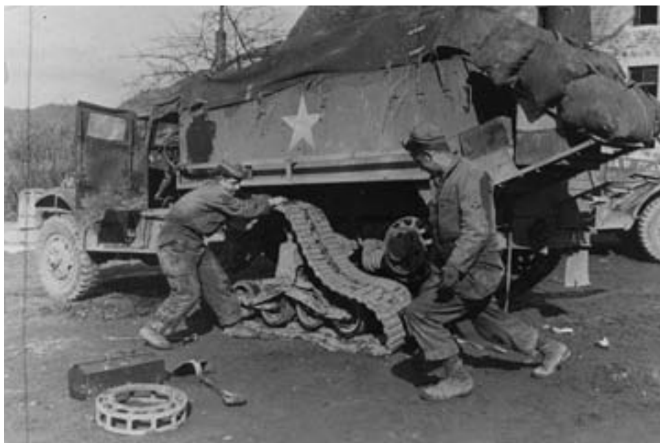
Track maintenance on a halftrack of the 9th Armored Division
