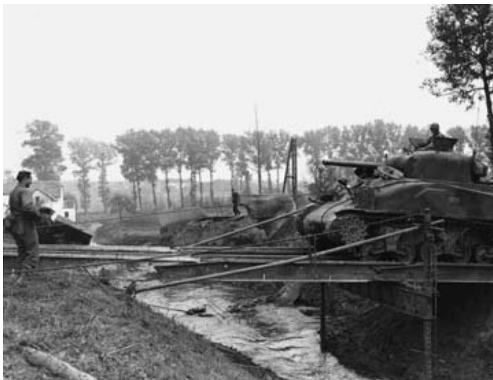
Tanks of the 66th Armored Regiment, 2d Armored Division, crossing an obstacle with the assistance of engineers
