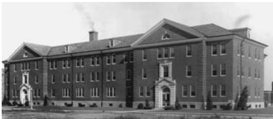
President Roosevelt's New Deal resulted in new facilities at Fort Knox during the 1930s, including the barracks pictured here.
